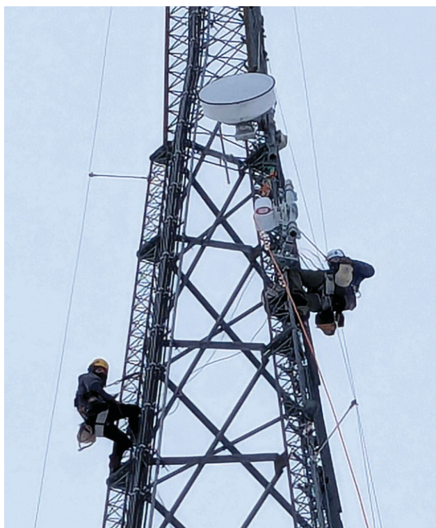
MARCS (Multi-Agency Radio Communication System) field engineers work on a tower that supports wireless digital communications for first responders and public safety officials.
